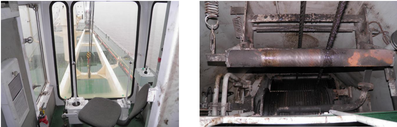
Figure 5: View of the inner and outer crane area from the position of the C/O.
